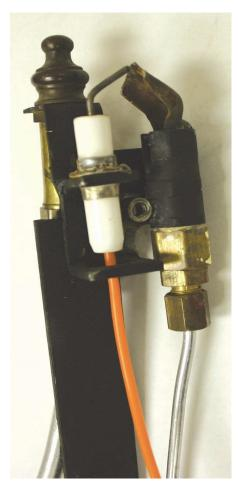
Check the Igniter/sensor ceramic for cracks. Also see to it that the ceramic assembly is fully seated in the bracket. For the best results, the igniter rod should be centered on the pilot hood and separated approximately 1/8"
