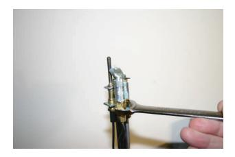
6 Reverse the procedure to reassemble the pilot burner using pipe thread to avoid gas leakage. Tighten all connections securely.
