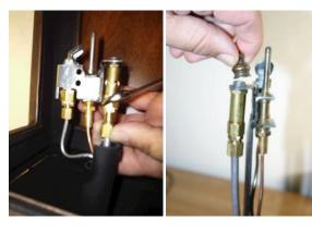
Remove the gas line from the bottom of the burner. Clean out the inside of the burner tube. After the unit is cooled down, remove the burner tip by using a pair of pliers as shown.
