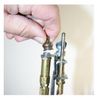
If the normal maintenance does not restore your flame to the proper height, please follow the next steps to clean the orifices inside the hurners.
